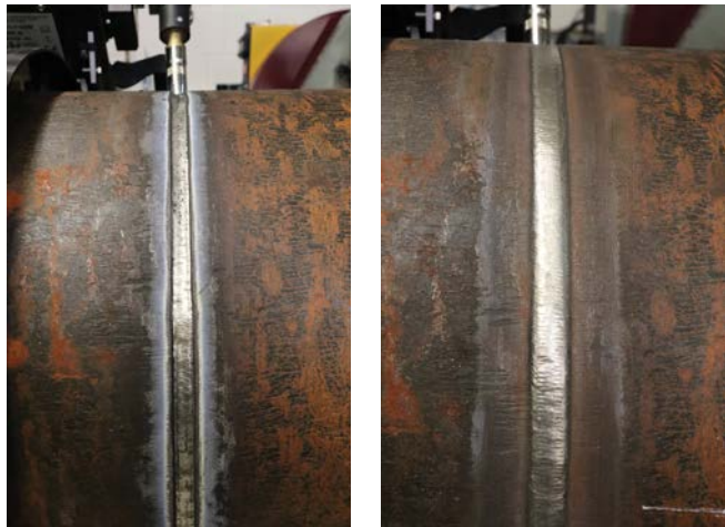
Weld bead appearance for the fill (left) and cap (right) passes completed using vaBW's pipeRunner® bug and band mechanised welding solution.
