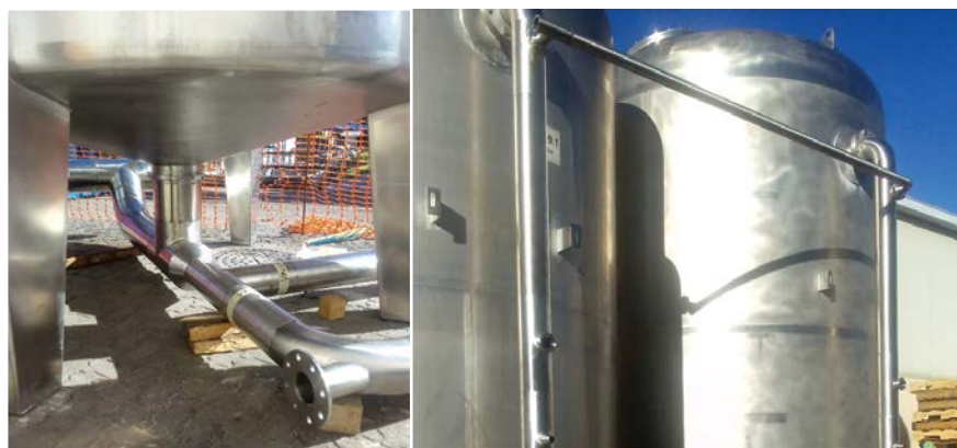
Carbon filters for AECI water at CERES Fruit Juices.
