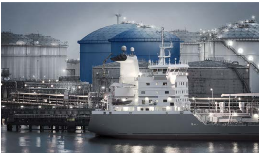
Current typical LNG gas storage tanks are able to contain more than 200 000 m 3 of liquefied gas.
