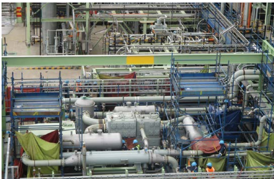
On Sasol's C3 polypropylene plant, Encore's mechanical fitters were responsible for installing and aligning equipment such as compressors and pumps, while the welding teams installed all the structural steel and piping.
