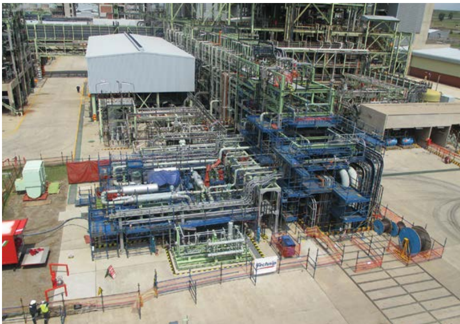
A notable project in Encore Engineering’s history was the Sasol’s C3 polypropylene plant expansion project at Secunda.
