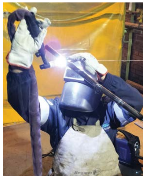
Encore Engineering Services has an elite group of GTAW welders to take care of small bore TIG welding.
