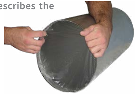
Figure 2: Soluble weld purge film being applied to a pipe end.
