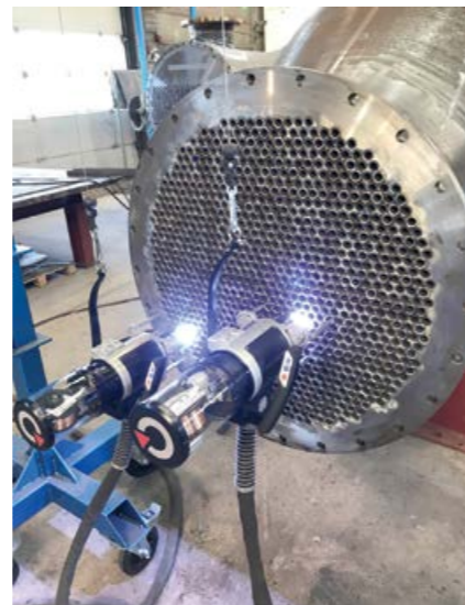
Efficient Engineering has purchased two state-of-the-art Polysoude orbital tube-to-tube sheet systems, which can each manage two independent welding heads.
