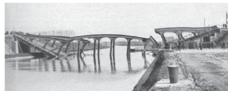
A 1934 image of a bridge collapse in Belgium that occurred while unloaded in the middle of a very cold night. "... if toughness is not present or has been degraded in service or the service temperature becomes lower than the values used in the design, then brittle fracture becomes a very real risk," Hobbacher advises.
